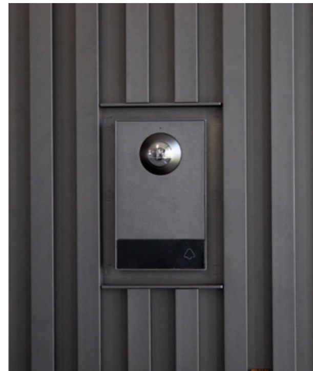
Video telephony is seamlessly integrated into the façade cladding with specially developed modules with blind plate in the same finish as the façade.
